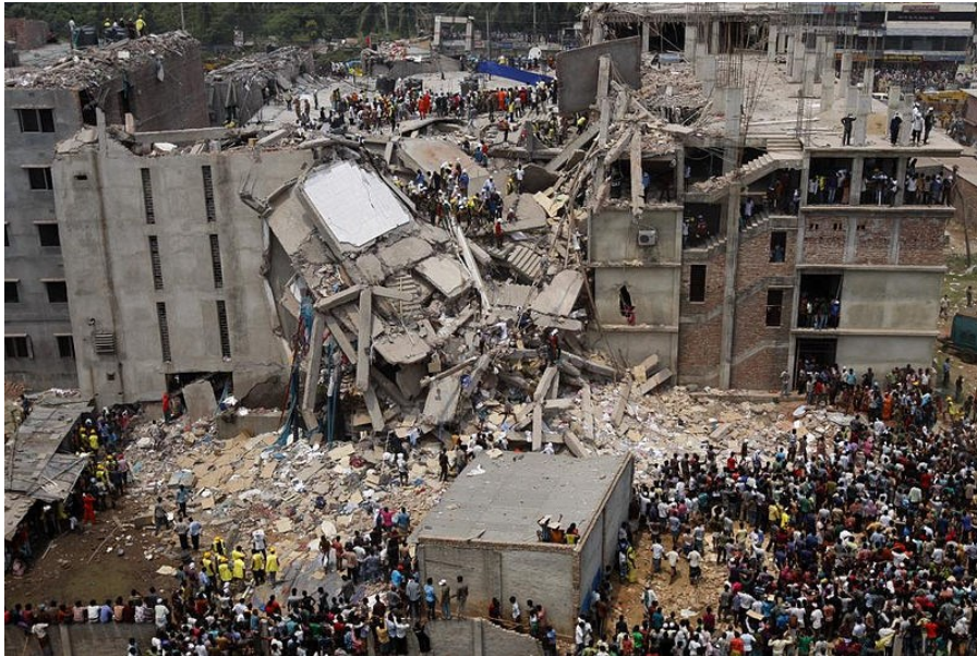
Figure 2. Aerial view of collapse.
